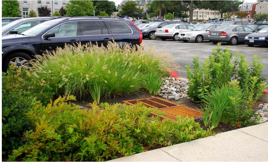
Example of a parking area rain garden
